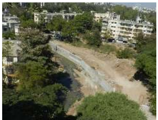
Wall being constructed along Ambil odha
